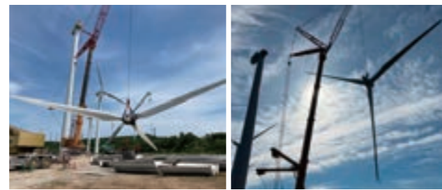
Dismantling wind turbines
