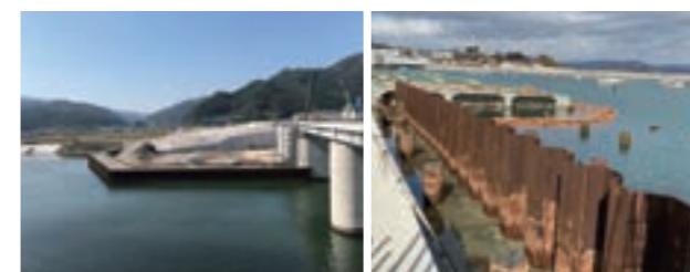
We delivered steel sheet piles needed at the bay construction sites along the Sanriku Coast, which was damaged by the Great East Japan Earthquake, and reused ones that were still valuable after use.
