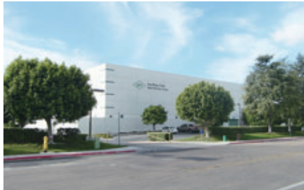
Exterior of the coil center
