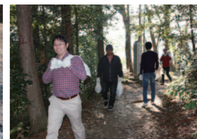
Volunteers carry sandbags to parts of the trail to be filled in
